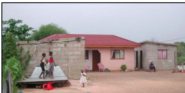
Plot with additional buildings in a low-income housing area in Gaborone, Botswana (photo: M Bourennane).
